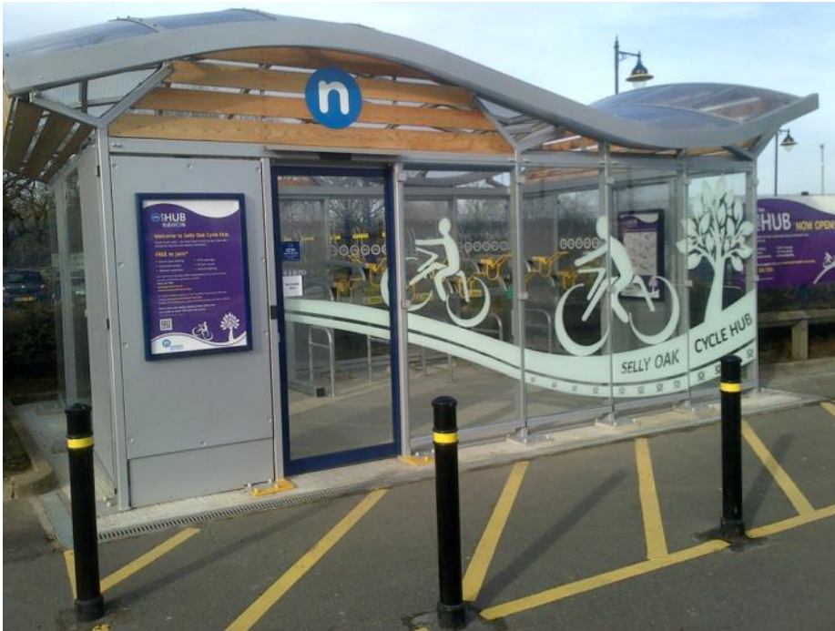
Unstaffed cycle hub at Selly Oak station has lighting, CCTV and smartcard secure entry.
