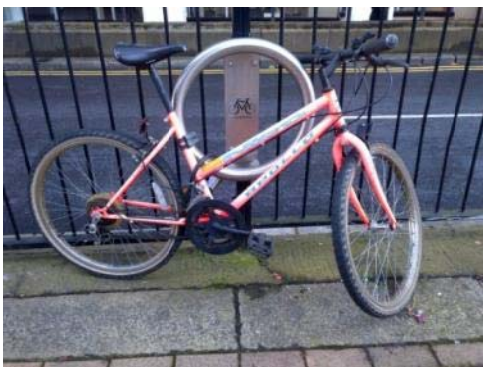
Retrofit parking hoop at Paradise Circus. This design can be fitted to existing guardrail, sign poles and other street furniture to offer more secure locking points.
