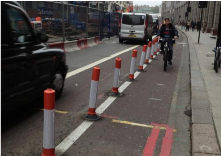
Temporary contraflow cycle lane during roadworks, London
