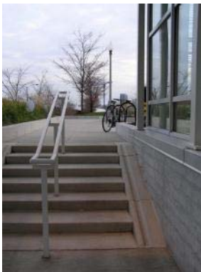
Simple concrete wheeling ramp to cycle parking at building entrance
