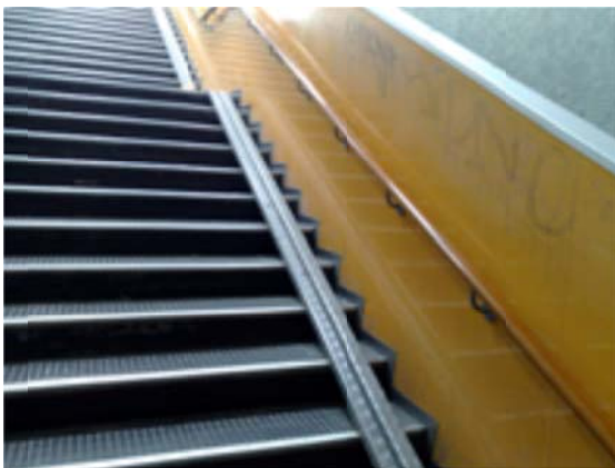
Typical ‘bolt on’ metal channel on railway footbridge
