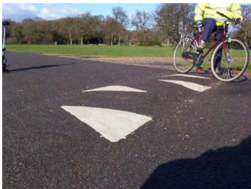
Speed hump at junction of footpath and shared path in a park.
