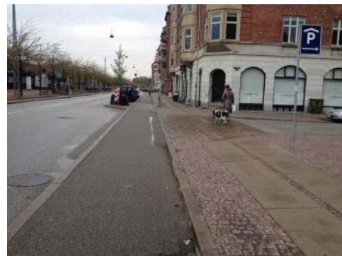
Side road is interrupted by a continuous cycle track and footway, vehicles using the side road are forced to give-way (similar to a residential driveway cross-over). Works for one-way or two-way cycling. May need yellow lining (or Diag 1026.1 marking for minor culs de sac) to prevent parking over junction mouth. (Phil Jones Associates)
