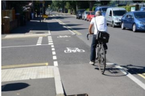
Brighton's Old Shoreham Road with-flow hybrid (half-height) cycle track (Alex Sully). Manchester's Oxford Road (right) has a higher demand for parking and an adjacent bus lane, therefore more signing and lining is required.
