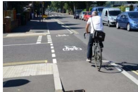
Cycle track crosses side road at carriageway level (Alex Sully). The cyclist here has the same status as if cycling along the carriageway (only works for one-way with-flow cycle tracks)
