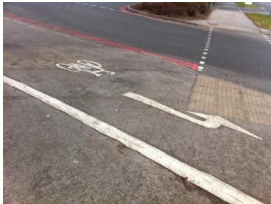
Use of Diag 1041.1 raised white line to separate space within a footway level cycle facility
