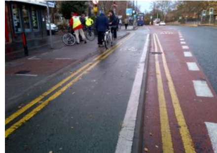
Brighton's Old Shoreham Road with-flow hybrid (half-height) cycle track (Alex Sully). Manchester's Oxford Road (right) has a higher demand for parking and an adjacent bus lane, therefore more signing and lining is required.
