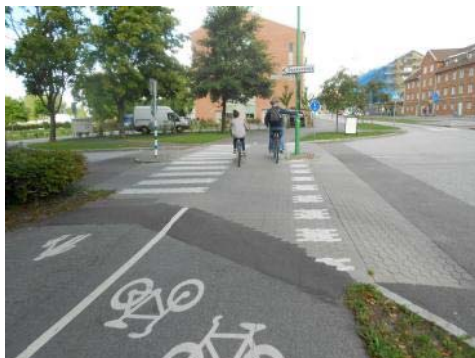
Cycle track crosses on a raised hump set back (at least 5.0m) from junction mouth (Phil Jones Associates). Cycle track uses 'give way' on raised flat top hump. Works for one-way or two-way cycling (can legally be done in UK using Give-Way markings, buff tactile paving and shared ped/cycle crossing area).
