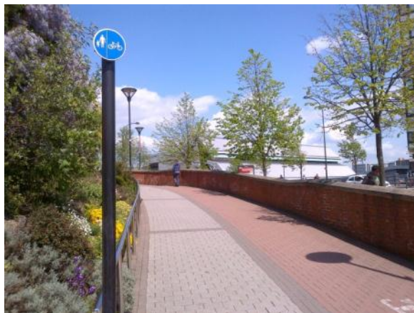
Different colour and texture separates pedestrian and cycle sides of footway helping to minimise signing and lining.
