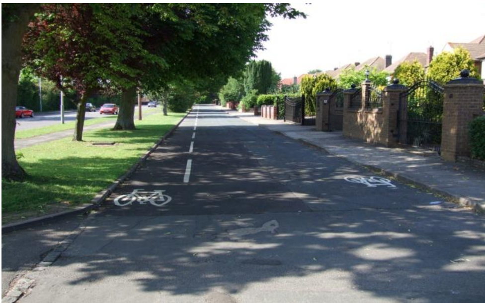
A cycle lane has been marked on the quiet side of this service road, while the cycle logo provides continuity on the side used for residential parking
