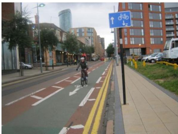
This contraflow cycle lane on Hurst St offers a good width and prominent markings including a buffer zone between oncoming traffic and the lane.
