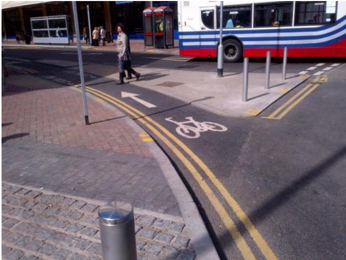
Entrance to contraflow lane at Corporation St is protected by a splitter island
