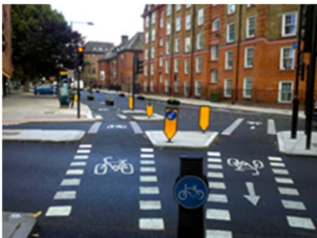
Where cyclists have a separate route marked through a signalled junction, elephants footprint markings will be authorised by DfT. (DfT)
