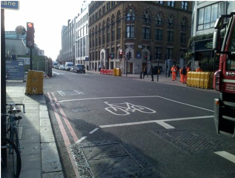
Advance stop line with Trixi mirror fitted to signal head
