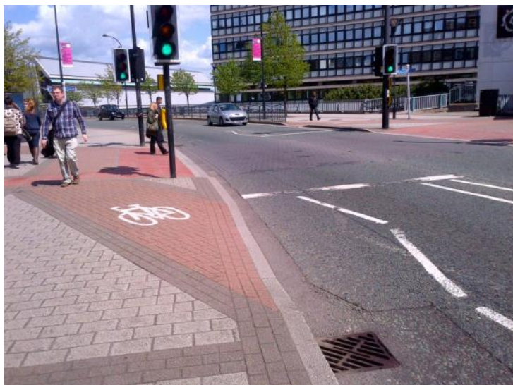
A simple 'jug handle' approach can be used to take cyclists from the carriageway into the waiting area of a toucan crossing.
