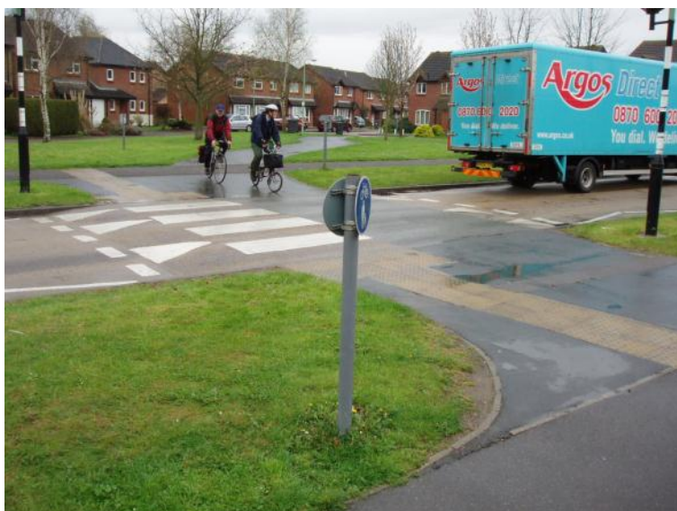
This example shows (currently illegal arrangement) a parallel cycle track and zebra crossing on a wide flat top speed hump. (Cycling England)
