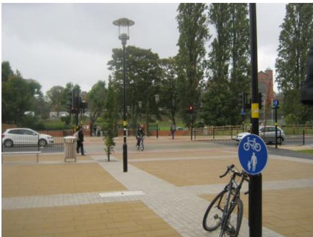
Wide toucan crossing with shared use approaches on A38 Bristol Road at Selly Oak
