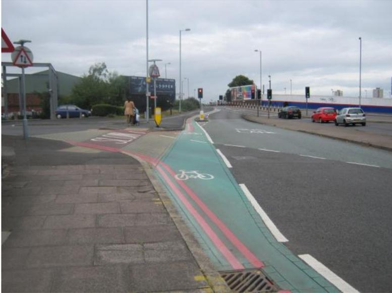
*This narrow cycle lane with drainage gully is uncomfortable and hazardous, placing cyclists too close to the kerb and potentially misleading drivers who will be turning left into the side road.*
