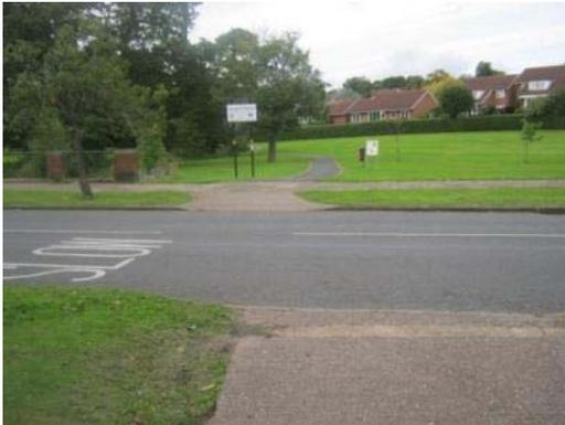
*On quieter routes such as this one in Bournville, provision of dropped kerbs may be adequate, while on busier routes additional half-size give way markings and buff tactile paving can be used to indicate a mid-block crossing point.*
