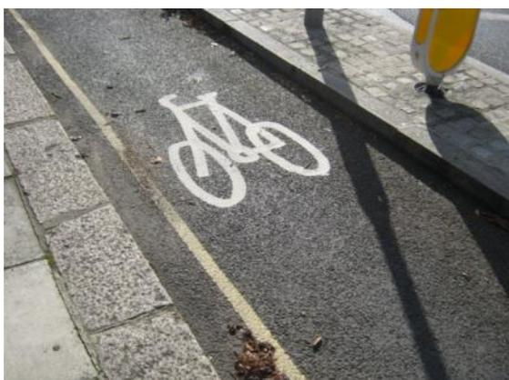
*Kerb separated cycle track width should be 2.0m to allow for sweeping and overtaking, chamfered kerbs would be more forgiving than right angled kerbs.*
