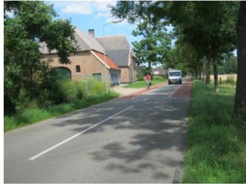
*Cycle lanes (or carriageway edge markings where the width is inadequate for lanes) may be used on low-flow suburban roads (<4000 vehicles per day) to change the 'feel' of the road to help reduce speeds. The residential parking on the left has been inset into bays in the footway to give a clear straight line to the cycle lane.*
