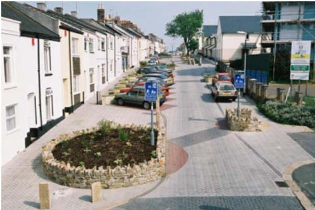
*Textured paving, narrow carriageway, greenery and limited forward visibility used to create low speed areas with priority for non-motorised users while retaining capacity of on-street residential parking. (DfT)*
