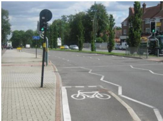
*Cycle track joining carriageway at a protected merge, joining a mandatory cycle lane after the crossing, Northfield.*
