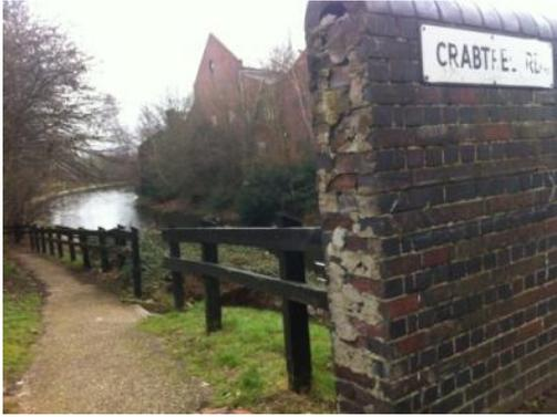
*Re-graded ramped access to Birmingham Canal Old Line towpath, sealed aggregate surface (but requires widening and removal of overhanging branches to bring up to cycle route standard)*
