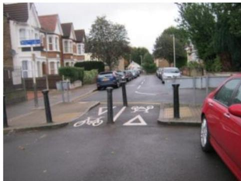
*Road closures (which may be for traffic/speed management or crime prevention, or to prevent traffic from using residential service roads) often make roads more attractive to cyclists due to the consequent reduction in traffic. Cycle 'gaps' at road closures offer 'filtered permeability' for cyclists where motorised through traffic is being restricted and should be incorporated into the design of all closures unless there is a safety issue.*
