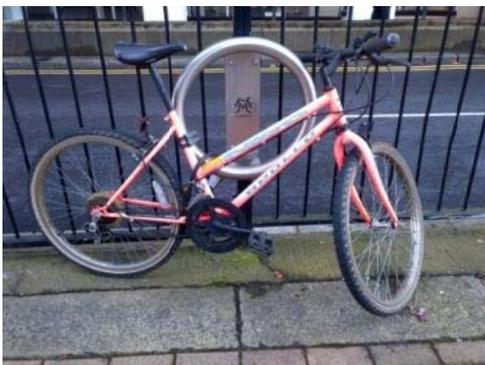
*Retrofit parking hoop at Paradise Circus. This design can be fitted to existing guardrail, sign poles and other street furniture to offer more secure locking points.*
