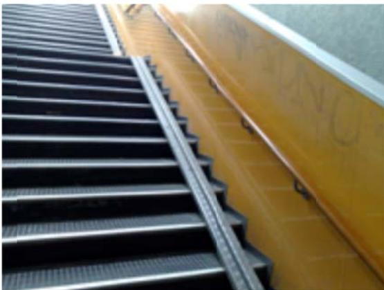
*Typical ‘bolt on’ metal channel on railway footbridge*
