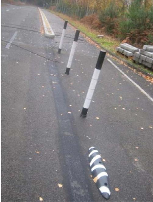
*TRL test site for separation using Zicla Zebra, Wand bollards, and kerb separation for a cycle track.*
