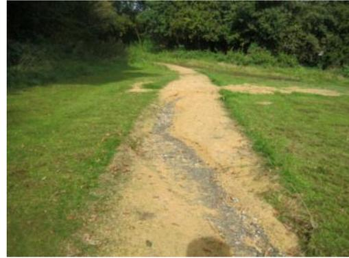
*Eroded gravel path on slope in Selly Oak Park. Sealed surface is more expensive but may have reduced overall costs when maintenance is considered*
