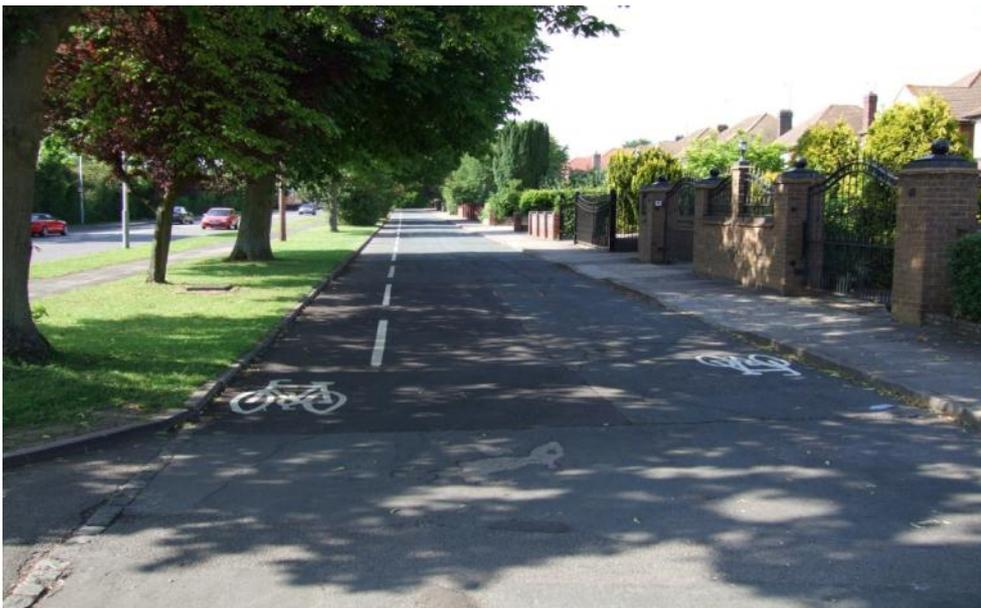
*A cycle lane has been marked on the quiet side of this service road, while the cycle logo provides continuity on the side used for residential parking*
