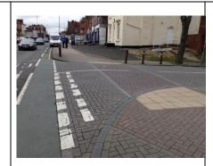
Junction entry treatments can take different forms but are used to help encourage all road users to negotiate junctions more slowly and carefully. They can incorporate different coloured surfacing and/or paving, raised sections of the road and changes to the road widths to reduce speeds.
