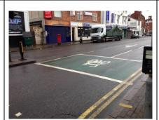
ASLs allow cyclists space to wait ahead of queuing traffic at traffic lights so that they are more visible to waiting traffic and can set off quickly ahead of traffic when the lights turn green.
