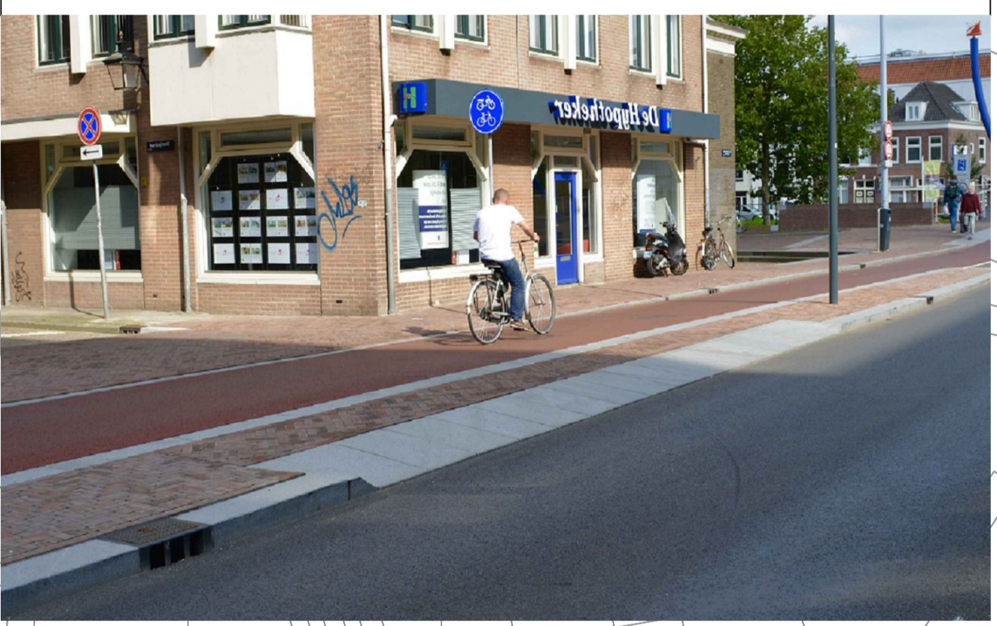
Inset D: Stepped footway / cycleway incorporating Dutch style kerbing
