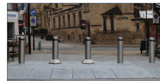
Hostile Vehicle Mitigation (HVM) with moving bollards for access.
