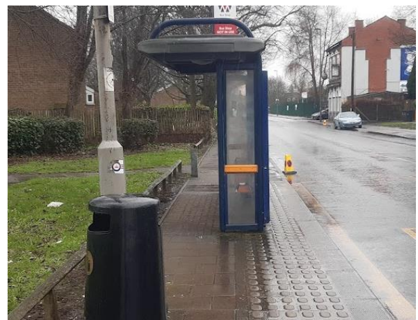
2.1 Junction of Cattell Road and Templefield St with poor dropped kerb position and drainage.
