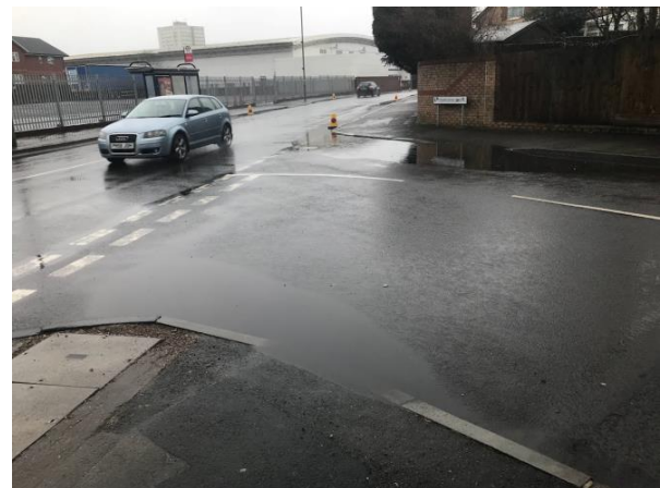
2.1 Junction of Cattell Road and Templefield St with poor dropped kerb position and drainage.
