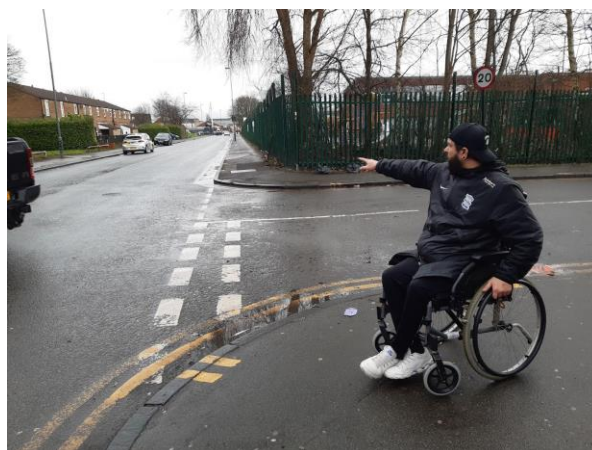
3.1 No dropped kerbs on Arsenal St junction
