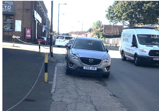
3.2 Damaged pavement surface and pavement parking
