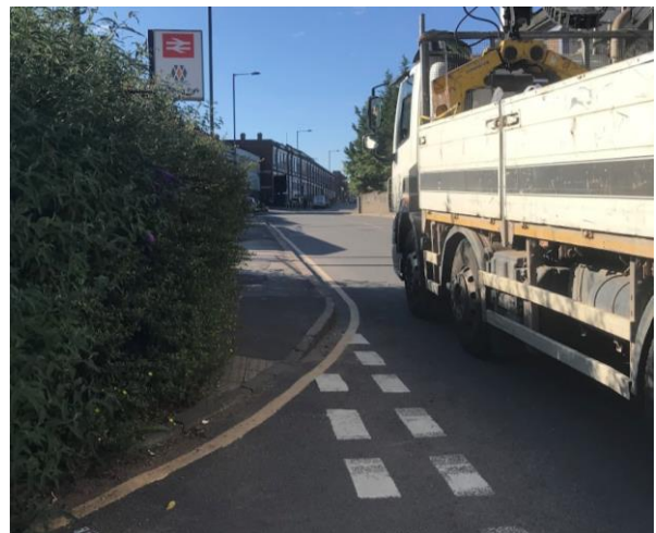
2.1 Overgrown pavement by entrance to Adderley Park station – tactile paving hardly visible
