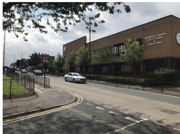
6.3 Girls' school with pedestrian crossing at end of Denbeigh St
