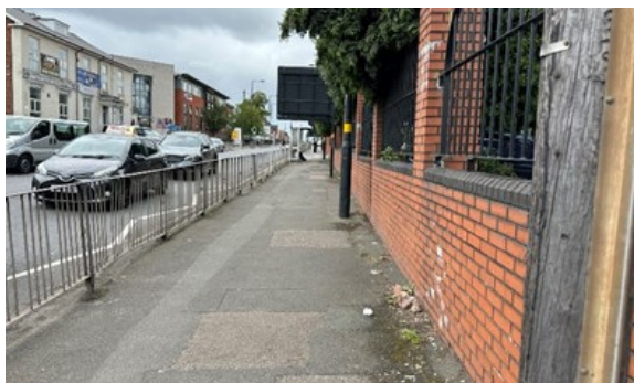
Declutter street furniture: Excessive guardrailing, Golden Hillock Road. Source: Pell Frischmann
