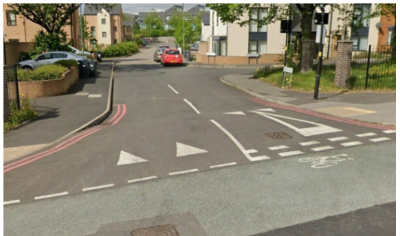
Example of a raised crossing at a side road. Source: Google Earth (2024)
