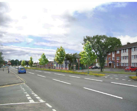
View after proposal looking East showing new mixed wild flower meadow and tree planting.
