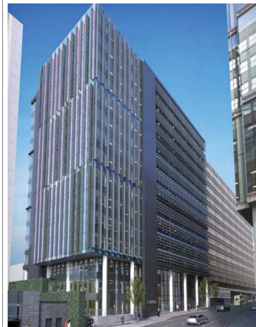
The Lumina development
