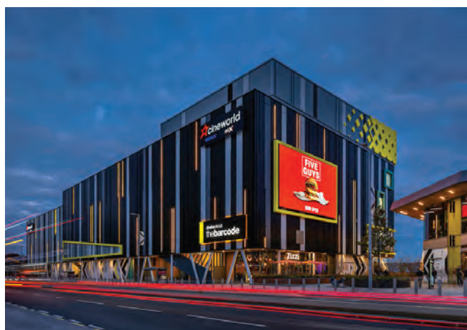
Barcode, Plymouth: purpose-built leisure attraction for the city centre including cinema, 'urban' golf, restaurants and car parking
