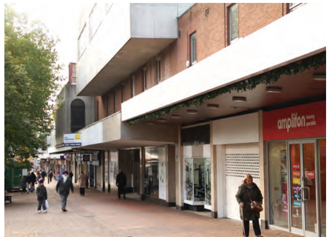
Gracechurch Centre's Parade frontage currently hosts some significant vacancies due to the loss of M&S and BHS.
