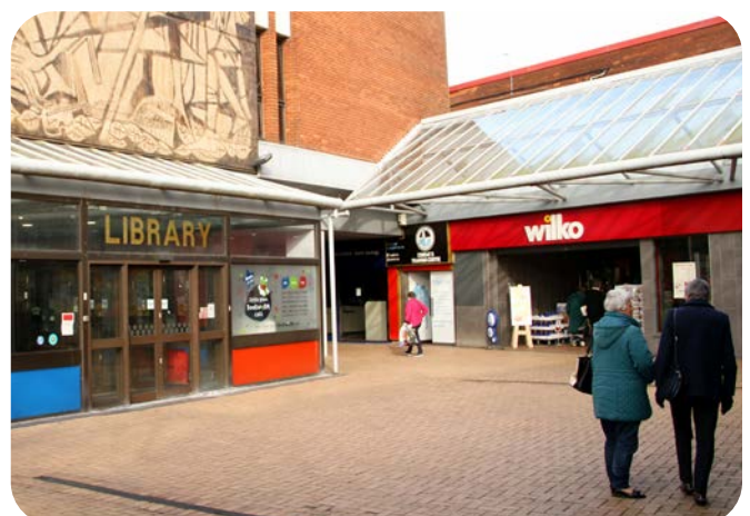
Reimagining Sutton Coldfield Library will be an important element of regenerating the town centre
