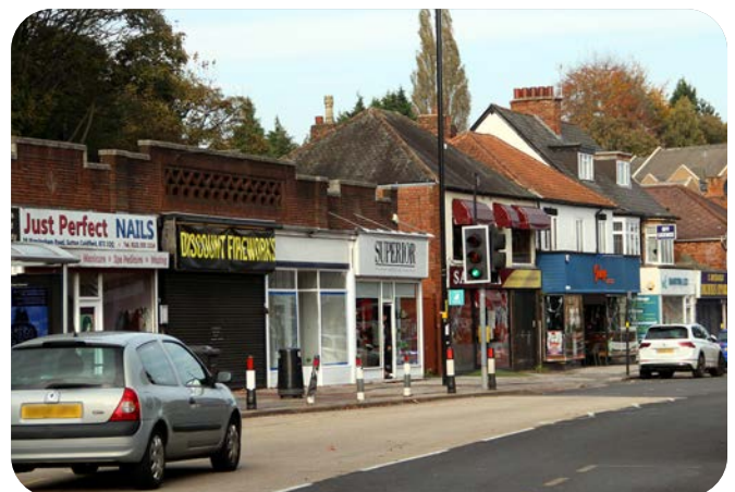
Some buildings along Birmingham Road are small in scale
