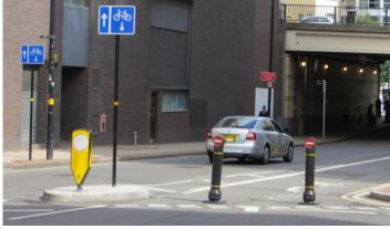
Advanced Stop Line – provides space at traffic signals for cyclists to wait ahead of queuing traffic where they are more visible to drivers and can set off quickly ahead of traffic when lights turn green.
