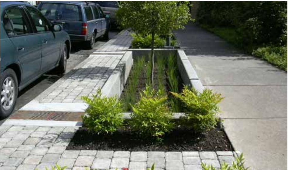
Figure 5.31 Example - Rain garden treatment along residential streets, 12 Avenue Green Street, Portland, USA
