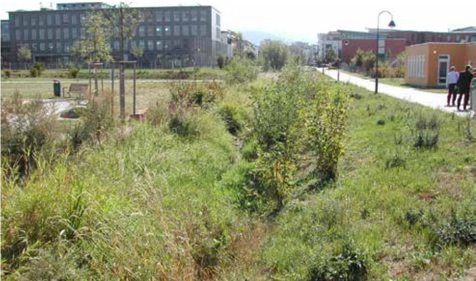
Figure 5.43 Convey swale with dense planting, Rieselfeld residential district, Freiburg, Germany
