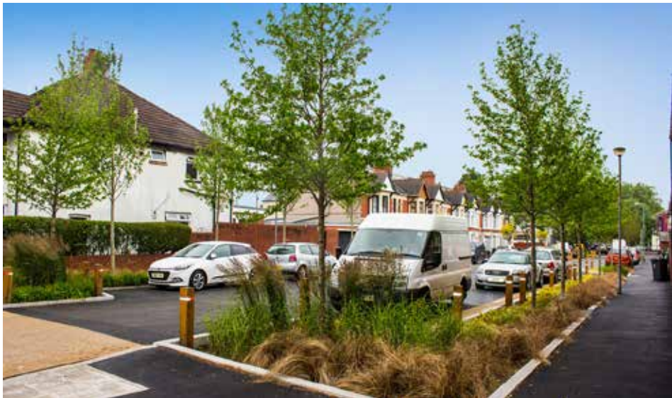
Figure 5.15 Example- Street Parking with rain garden, Greener Grangetown, Cardiff, Wales
