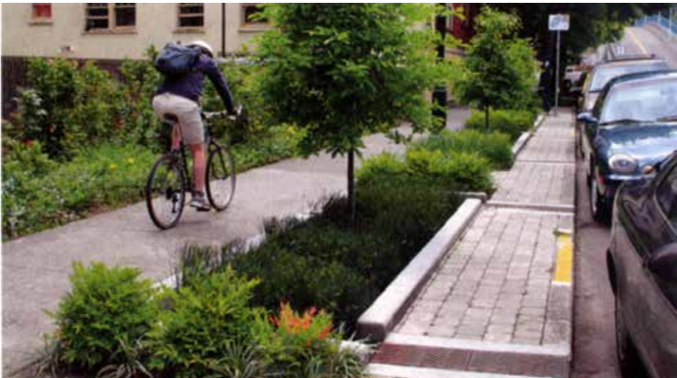
Figure 5.46 Example - Street rain garden treatment, 12 Avenue Green Street, Portland, USA
