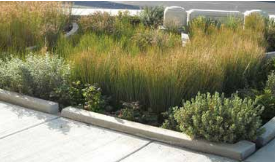
Figure 5.30 Example - Dense planting on side street for drainage attenuation, Sandy Boulevard, Portland, USA
