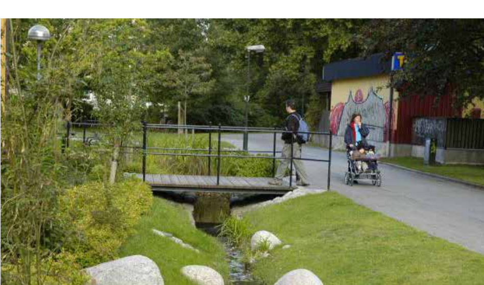
Figure 5.44 Example -Conveying swale with crossing bridge, Malmö, Sweden
