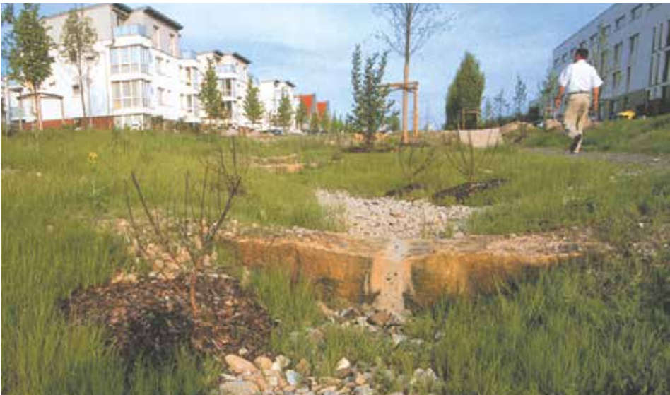
Figure 5.42 Example -Dry bed SuDS treatment, Kronsberg Hannover (part of expo 2000), Germany
