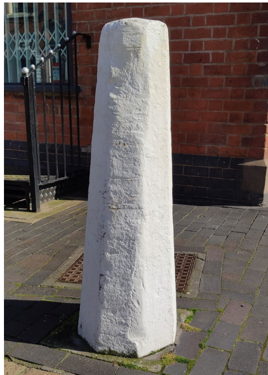
Image: Sandstone bollard (now painted), blue brick paviors, pink granite kerb, Vyse St
