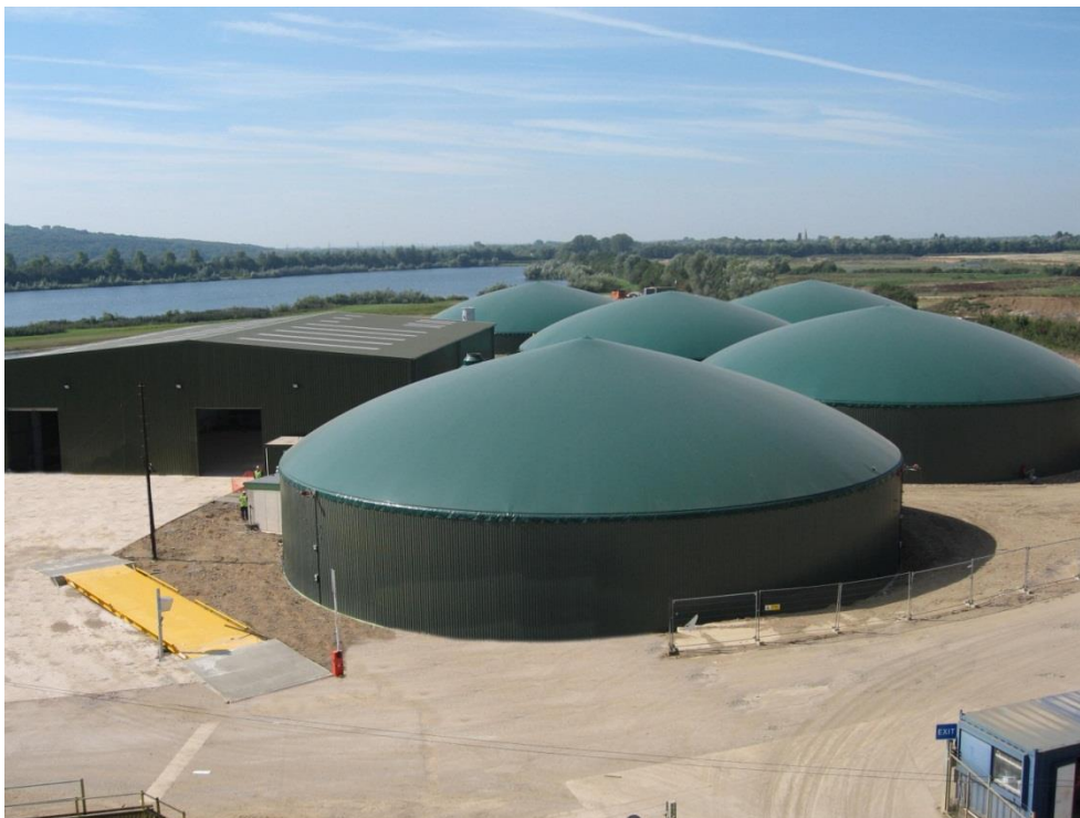
Agrivert Cassington Anaerobic Digestion facility, Oxfordshire, UK, www.biogas.org.uk
