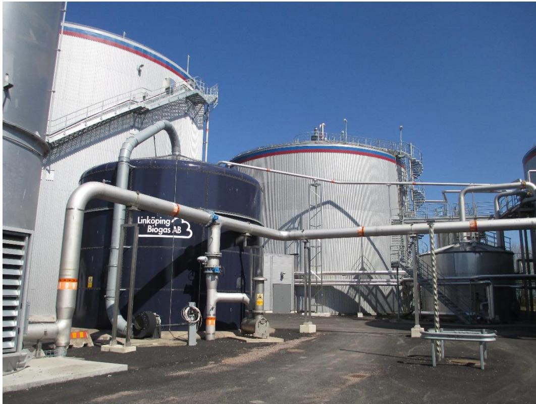
Linköping Biogas to vehicle fuel plant, Sweden
