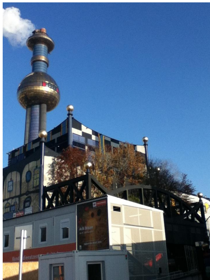
Spittelau EfW facility, Vienna, Austria
