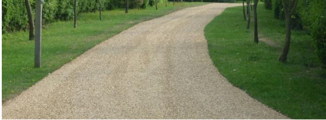
Tar Spray and Chip Surface Dressing
