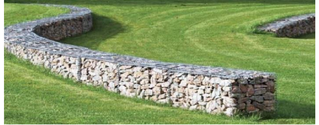
Curved Gabion Retaining Walls
