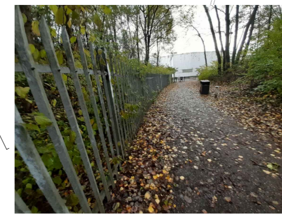
Remove the end panel from the existing palasade fence to allow access to the woodland
