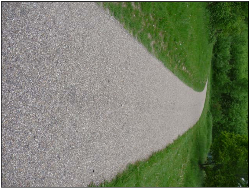
Example of a bitmac (tarmac) path with a bounded gravel surface dressing
